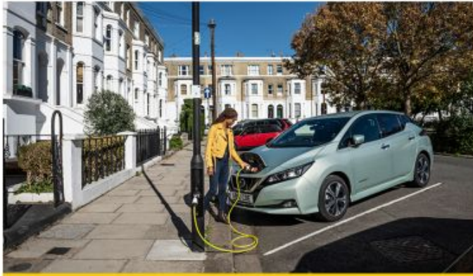
Shell's ubitricity provides on-street charging for electric vehicles through lamp posts across the UK and the European Union.
