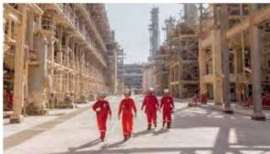
Operates at Pearl GTL plant, Qatar.
