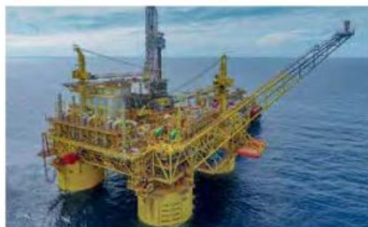
Malikai deep-water platform, Malaysia.
