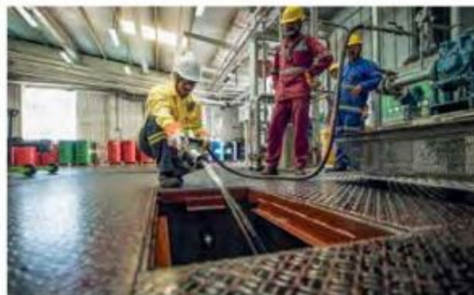
Shell lubricant plant, Oman.
