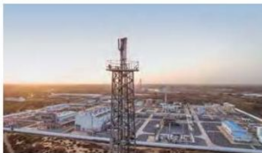
Changbai Natural Gas Processing Facility China.
