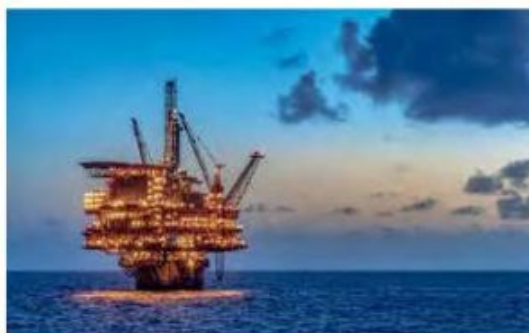
Perdido offshore deep-water platform in the Gulf of Mexico.
