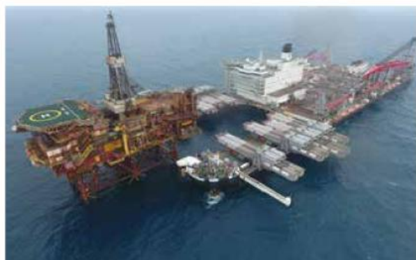
The Pioneering Spirit vessel has now lifted and removed the topsides of Brent Alpha, Brent Bravo and Brent Delta.
